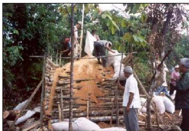
Phot 2. Sawdust mould kiln
