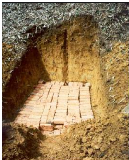
Phot 4. Modified earth pit kiln (Brick floor)
