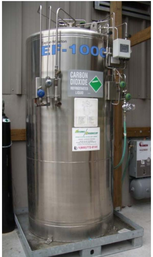
**CO<sub>2</sub> Supply System for Algae Pilot Plant**
